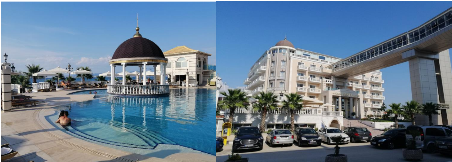
SANTA BEACH HOTEL KOMPLEX
